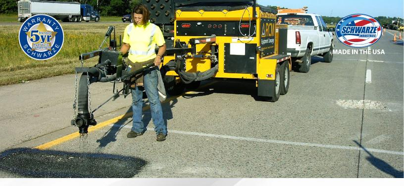
A recent report by the Minnesota Department of Transportation conducted a present worth analysis of spray patching vs. traditional "throw and roll" and found the cost of spray patching to be 1/3 the cost (\$2.31 per patch vs. \$7.17 per patch), again due to lower labor and the fact that spray injection lasted 4 years compared to throw and roll patches having to be refilled annually due to wash out from weather.
